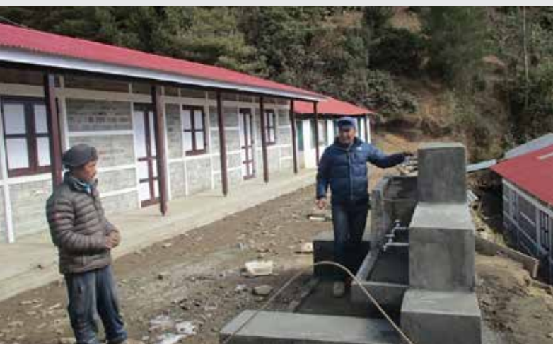
New water supply and classrooms at Pike school.
