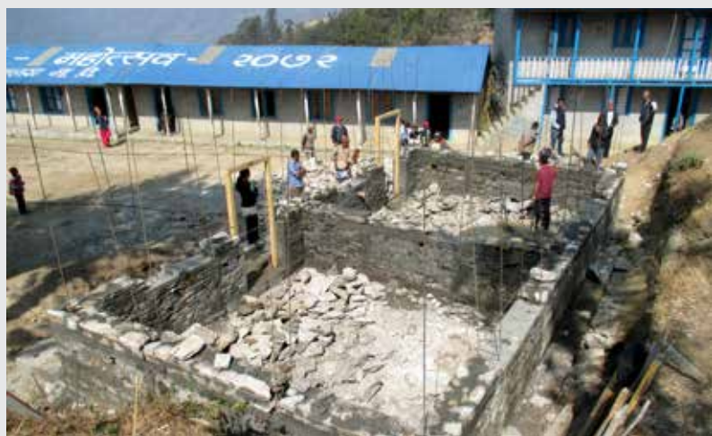
Work in progress at Himalaya Secondary School, Jubu.
