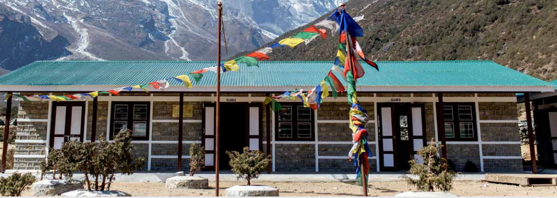
New earthquake-strengthened classroom block at Thame school.
