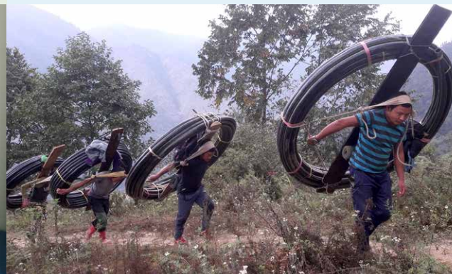
Workers installing pipelines in the Solukhumbu District.
